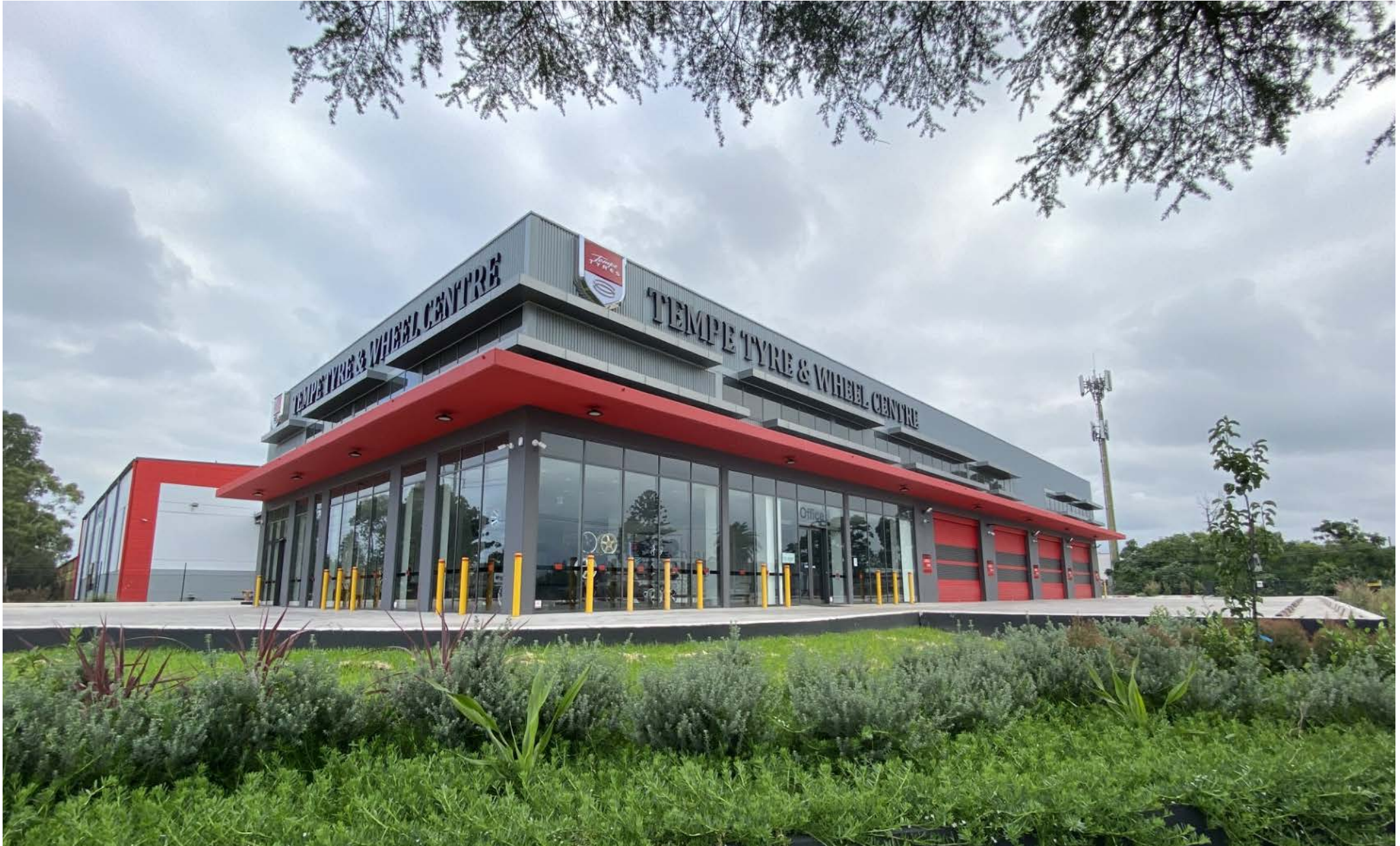
Tempe Tyres, 2072-2074 Castlereagh road Penrith Completion 2021 Value $9.5 million
