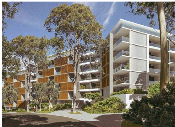
6-16 Hargraves Street - Gosford Constructed 2019 Type: 8 Storey x 93 Apartments Project Cost: $29,500,000
