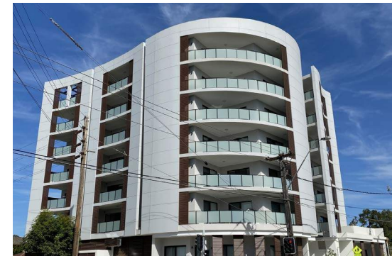
114-116 Station Street, Penrith Constructed - 2017 Type: 7 Storey x 45 Apartments Project Cost: $21,000,000
